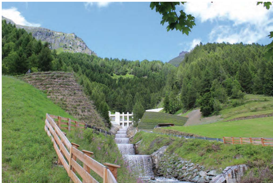
Figure 14: Technical measure for protection of debris flow above the village of Prägraten ( Peter Hajek ).
