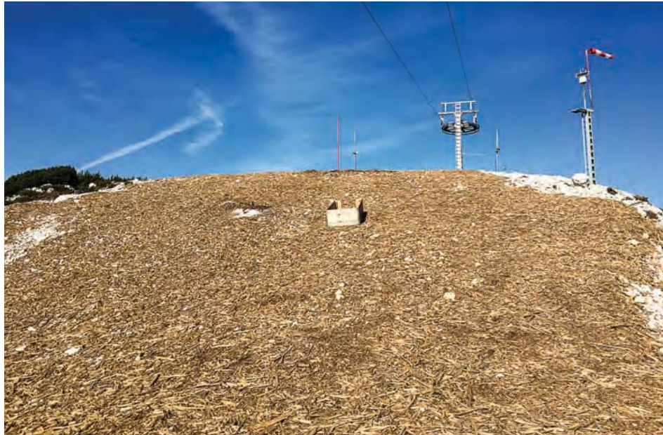
Figure 57 : Covering a ski slope that is almost without soil with wood-chips – an initial activity towards gradual restoration of grass cover; Vogel ski area.
